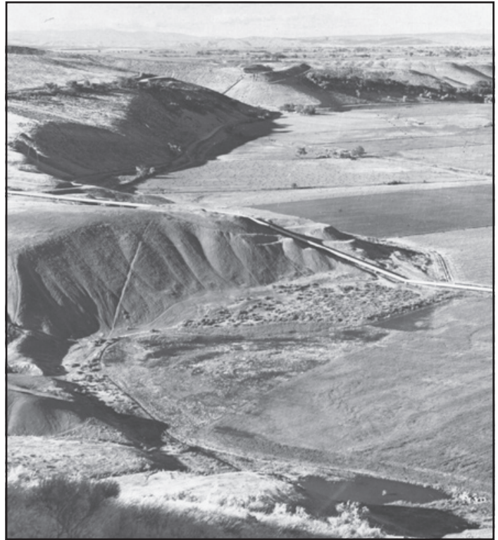
The Owyhee or Malheur Siphon carries irrigation water to benchland off the valley floor.
